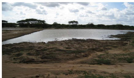
Figure 3: Trapezoidal bund in Wayu after first rain (November, 2008)
