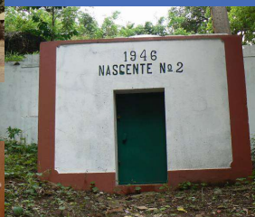
Rehabilitation of Boma Spring
