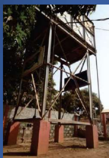
Elevated Reservoir of Bairro 4
