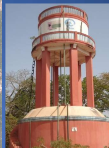
Elevated Reservoir of Boma and ground level reservoir of Praça
