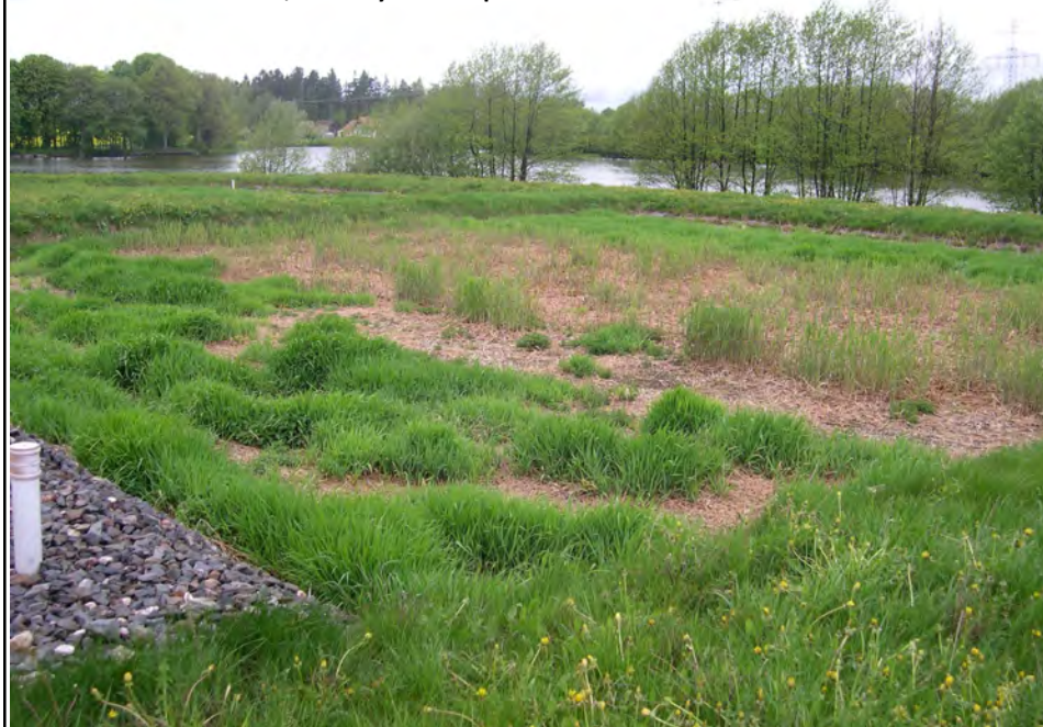
HF CW Zbenice in 2004, after 7 years of operation
